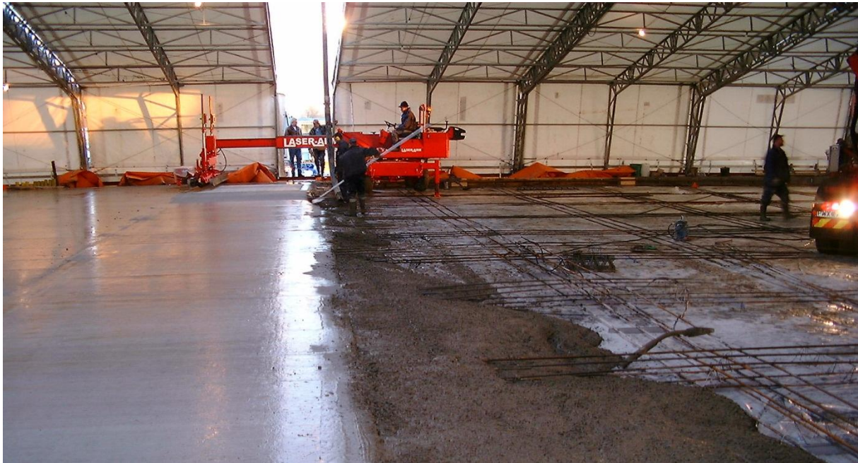
Figure 2.5: Typical semi-automation of concreting of piles supported SFC floor slab with combined reinforcement in strips. In this sequence the laser-screeder is equipped with topping spreader. Still people must run the machines and bull-float and power floating the surface. Photo: Hedebratt (2001).
