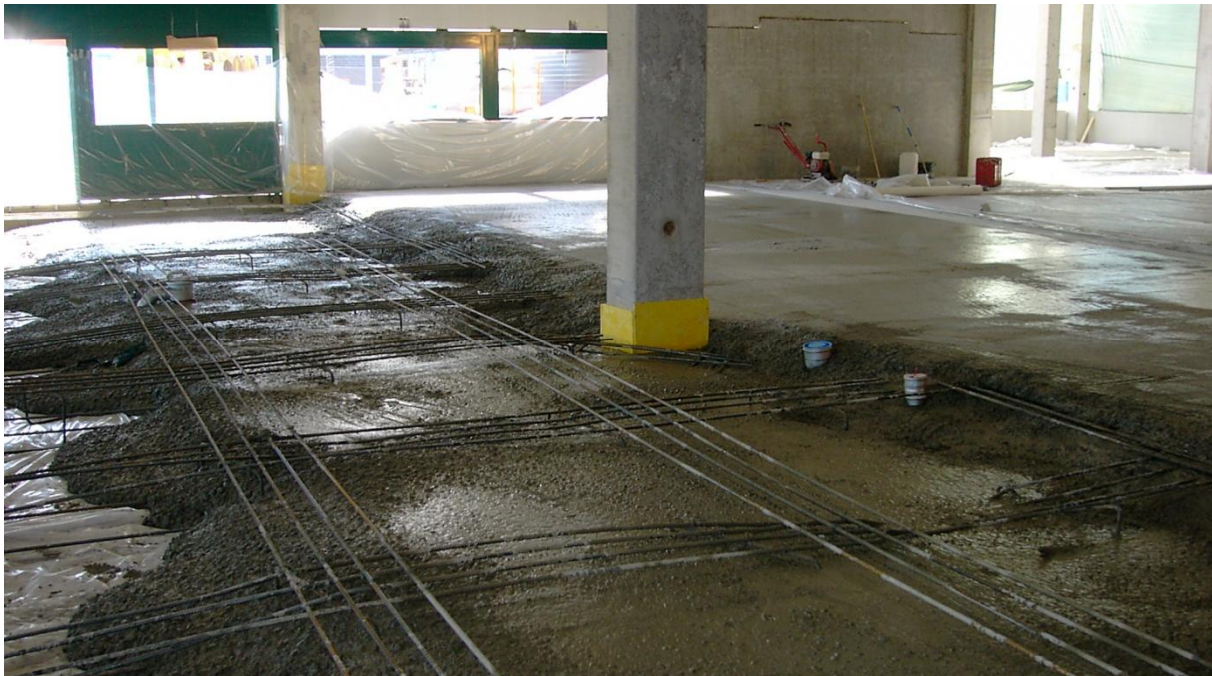
Figure 3.4: The top layer of reinforcement bars in project No. 9 (from Paper B ).
