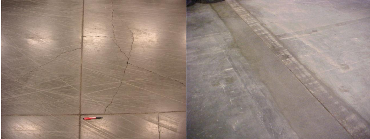
Figure 4.1: Recurrent damages in investigated floors. To the left curling and cracking near joints and at corners. To the right curling that has been grinded ones and later levelled with topping screed. From Paper A .
