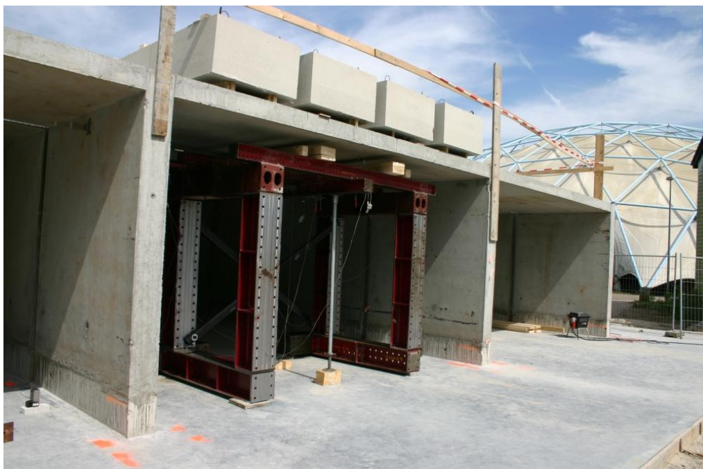
Figure 3.22: Loading of slab. Photo: Anne Hoekstra (2011).
