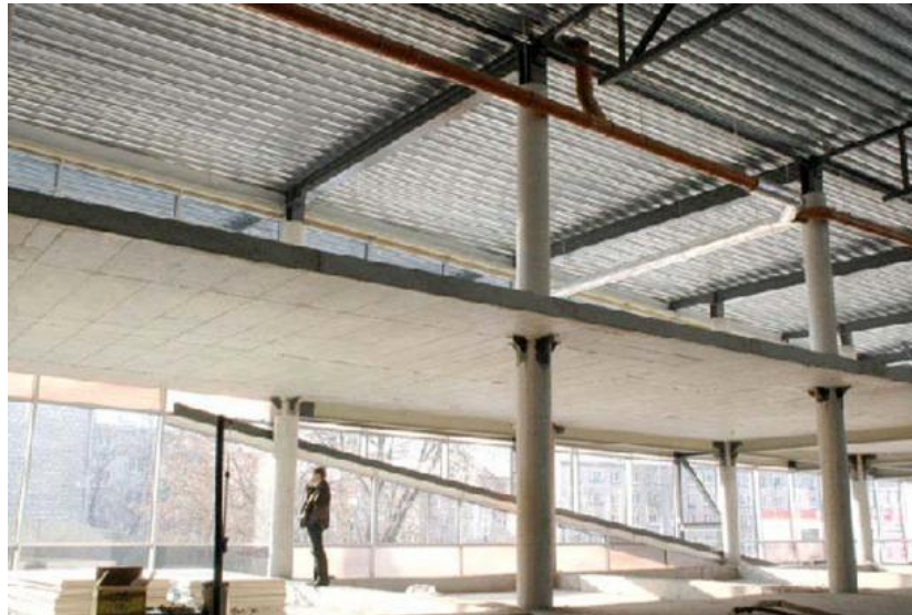
Figure 3.21: These flat slabs in several levels, was loaded with “service load”. (Destrée & Mandle, 2008).
